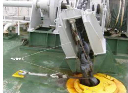
Picture 2 showing Securing Wires Courtesy TE Subcom
